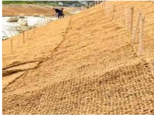
Figure 2. Biodegradable soil erosion control mat [45].
